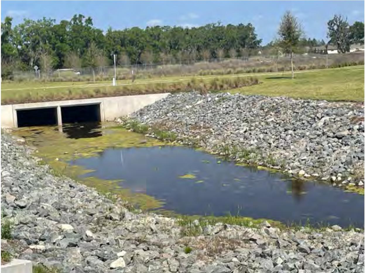
The rock basin has filamentous algae within it. The D.M. has contacted the pond vendor to include this basin in the contract.
